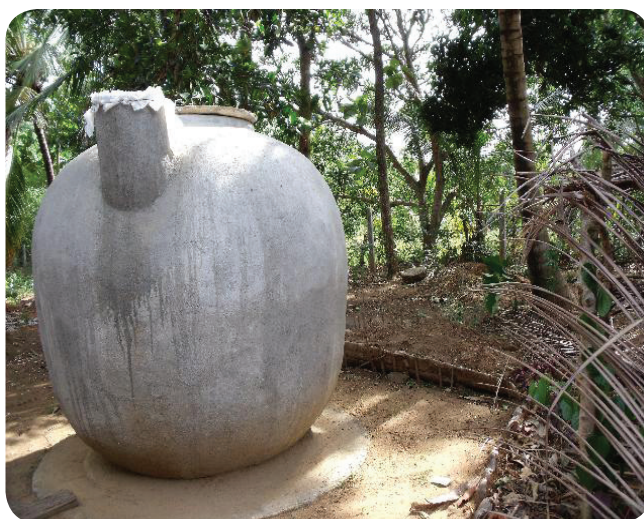
rain water tank
